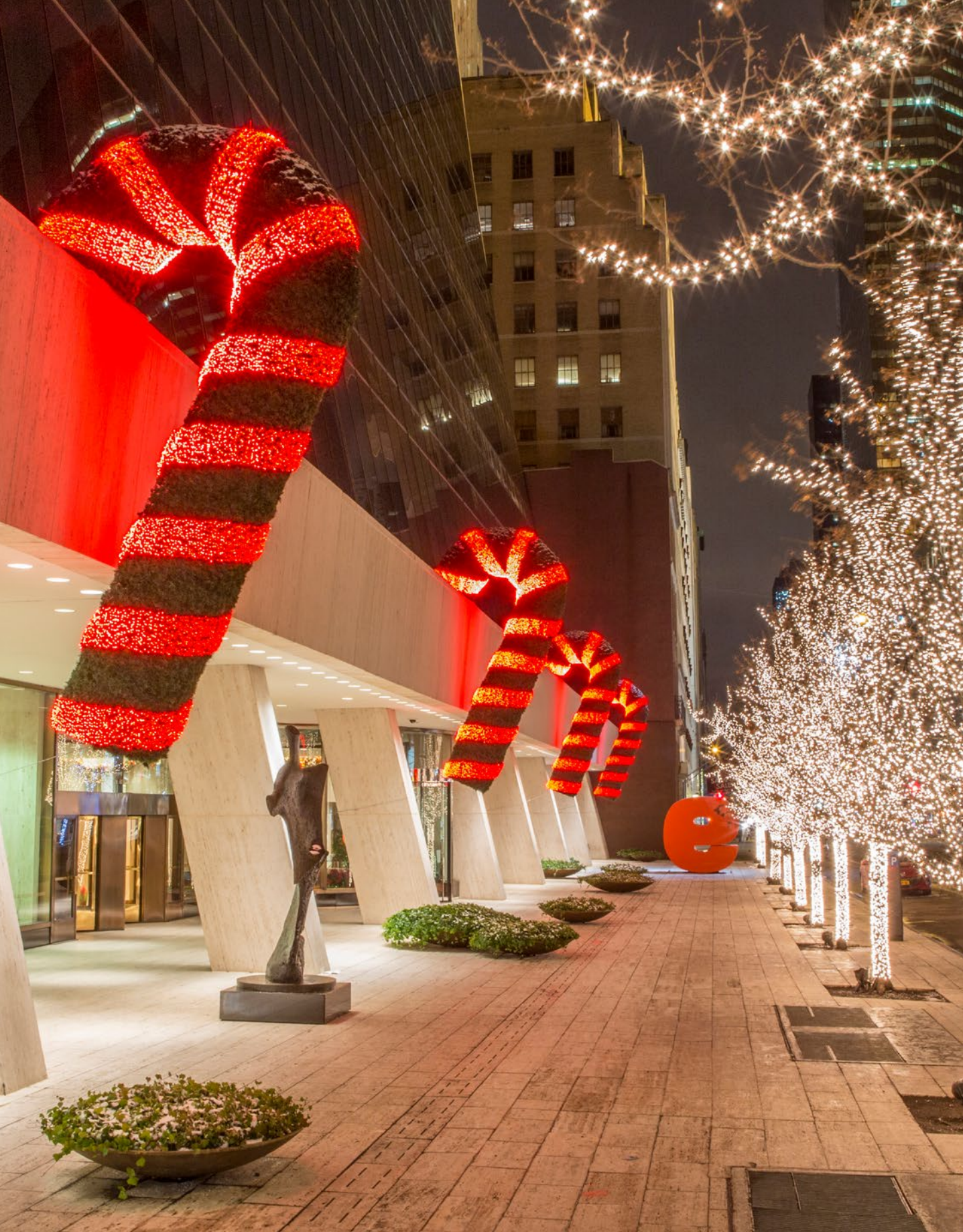
The Solow Building, New York – USA
